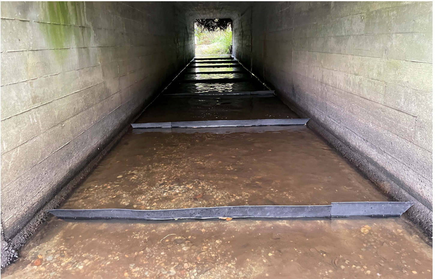
Another Flexi Baffle installed in a culvert.
