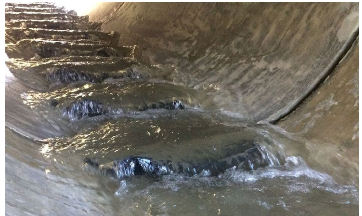
One benefit of a flexible baffle such as the Flexi Baffle is that it bends over in high water and does not catch debris.
